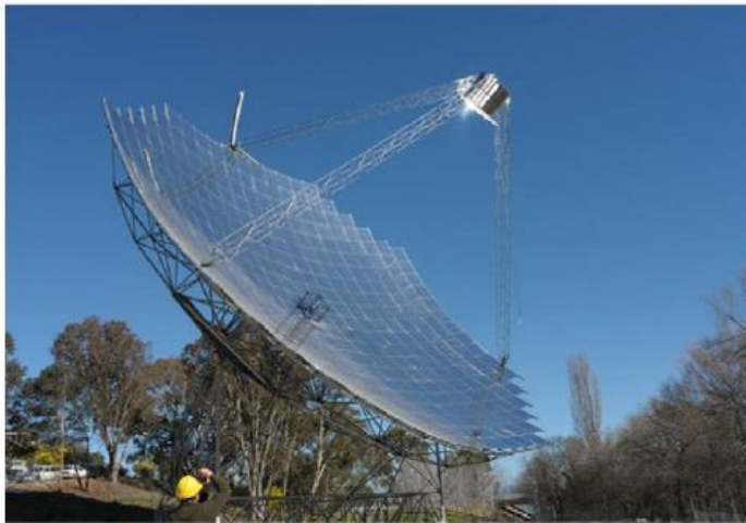
Fig.1 Parabolic Dish Type solar collector
